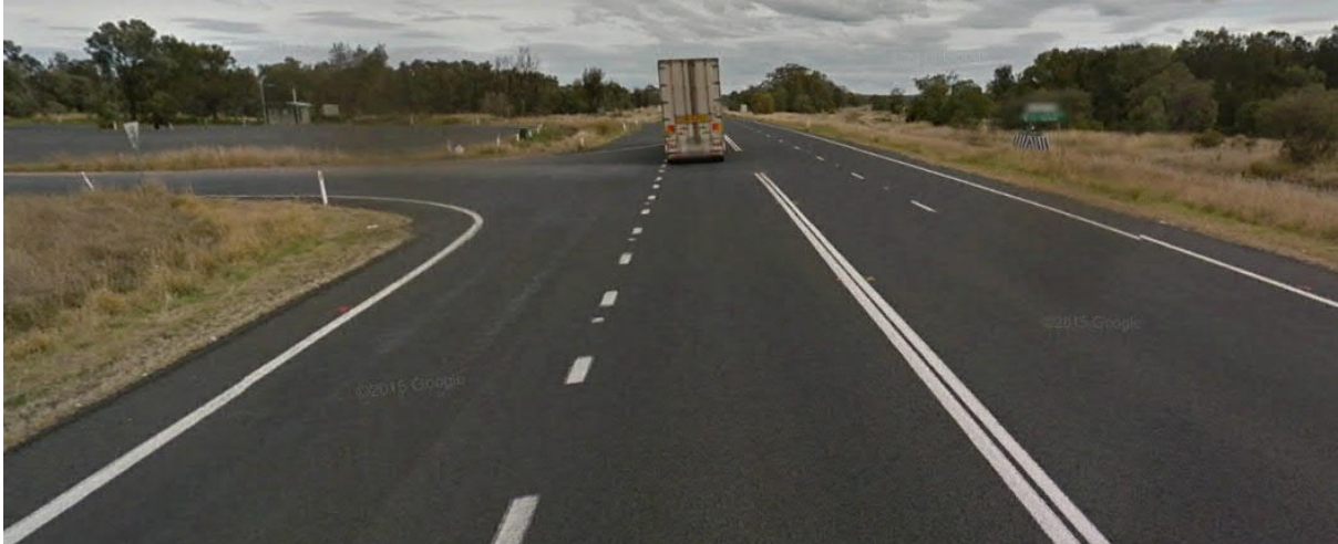
Figure 2: IB Bore Road - Newell Highway Intersection looking south
